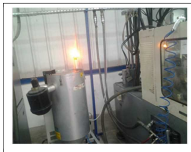
Figure 9. Implementation of poka-yoke: Sensor with alarm.
